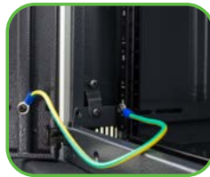
Front and rear doors equipped with ground wires
